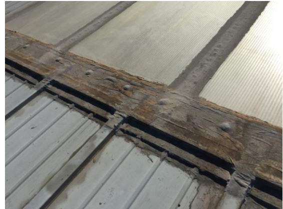
Detall remat claraboies a reparar
